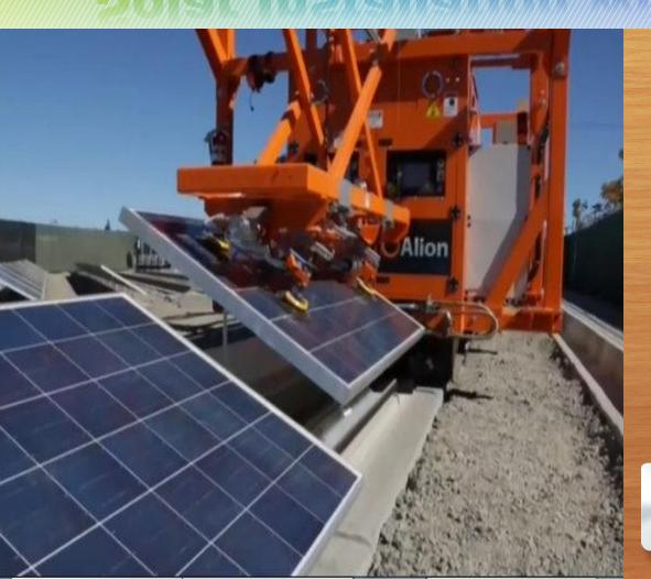
Alion Energy, has developed a new automated system that is seven times faster than conventional solar installation.
